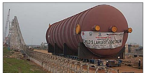
World's largest Coke Drum was erected at Paradip Refinery site. The Coking Unit will produce raw petroleum coke. The coke drum weighs 630 MT and is 45.52 meter tall and has 10.67 meter diameter. Rajkumar Ghosh, Director (Refineries) complimented IndianOil employees for tirelessly working to accomplish this gigantic task. The Rs.30,000 cr project of IndianOil will change the skyline of the region, once completed, said Ghosh.
